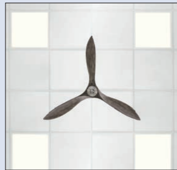
Fig. 9: Especially at workplaces, the flickering of ceiling fan blades running through the lighting is disturbing. This should be taken into account during planning.
