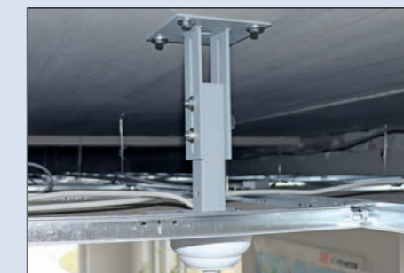
Fig. 4: Trimming support SST
